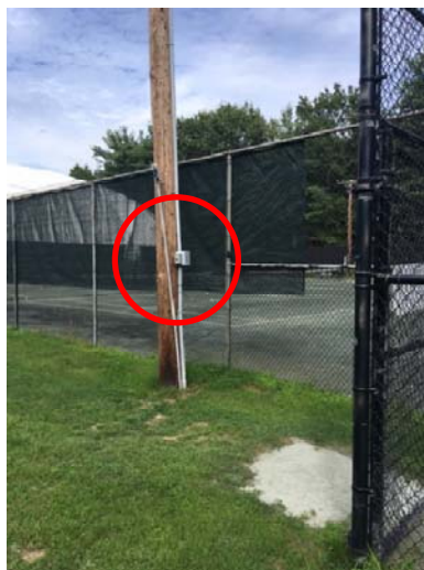
Light switch for Court C
