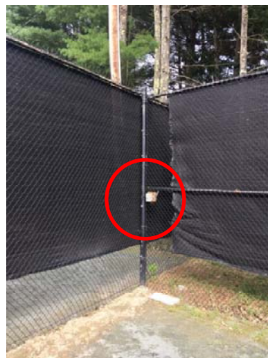
Light switch for Court D
